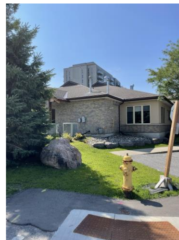
Photo 10 - River Parkway Children's Centre. Taken from Phase One Property, facing southwest
