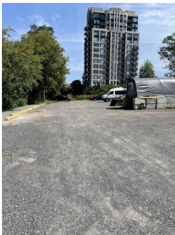
Photo 3 - Gravel parking area at southern portion of Site. Former railway corridor, facing east.
