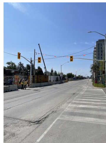
Photo 12 - Light Rail Transit construction south of Richmond Rd. Facing southwest.
