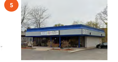
797 RICHMOND RD. EXISTING 1-STORY DENTAL OFFICE
