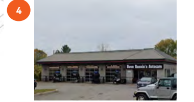
801 RICHMOND RD. EXISTING 1-STORY AUTO SHOP
