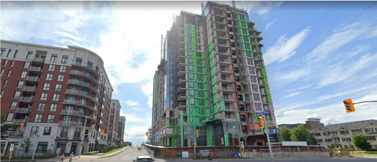
Under construction Haven Towers on Marketplace Avenue, looking west
