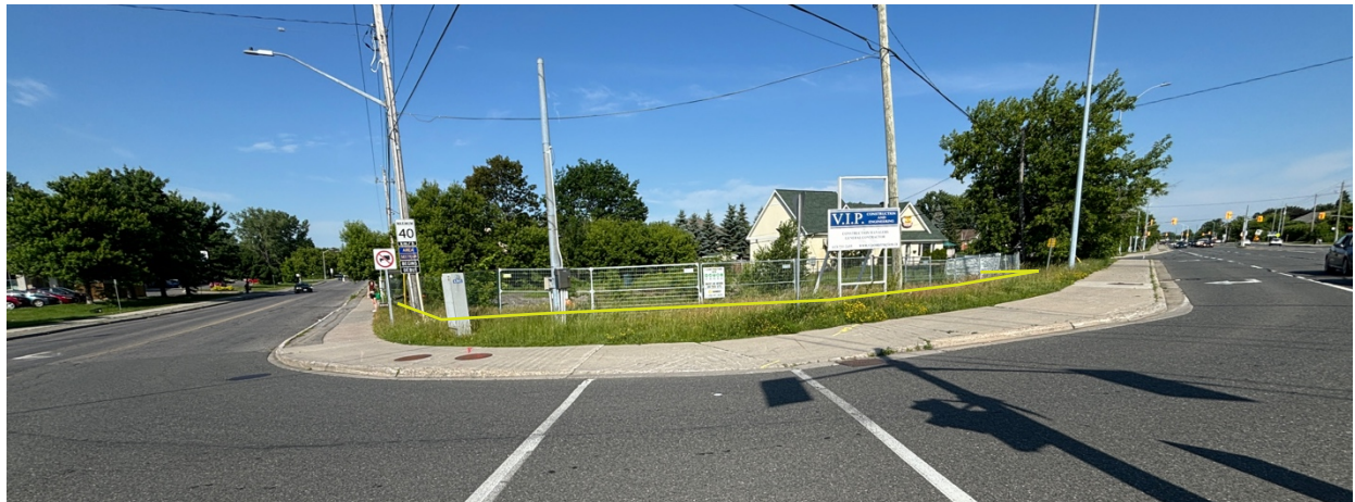
Figure 2: View of subject site from the corner of Queensdale and Bank
