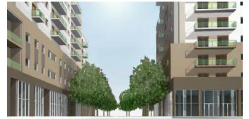
ACCESS BETWEEN BUILDINGS B AND C
