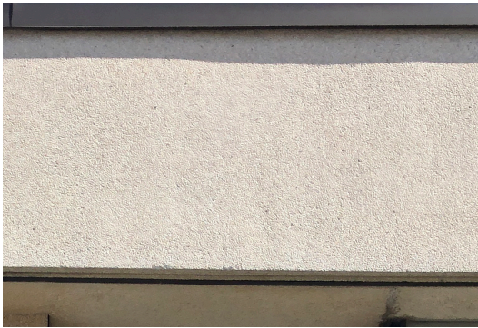
Figure 23. Aggregate-faced concrete paneling (ERA, 2021).
