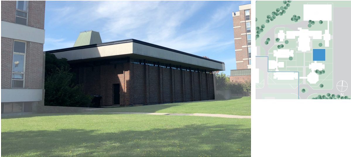
Figure 5. Building D, viewed from southeast (ERA, 2021).
