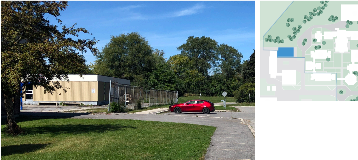
Figure 11. Building N, viewed from south-east (ERA, 2021).
