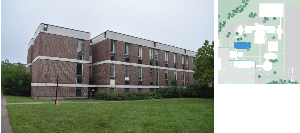
Figure 9. Building J, from Sisters' courtyard (ERA, 2021).
