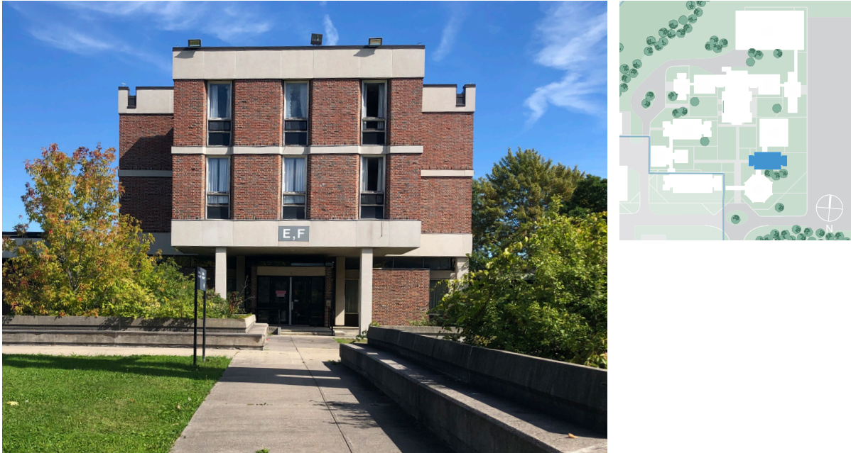
Figure 6. Building E, west elevation (ERA, 2021).
