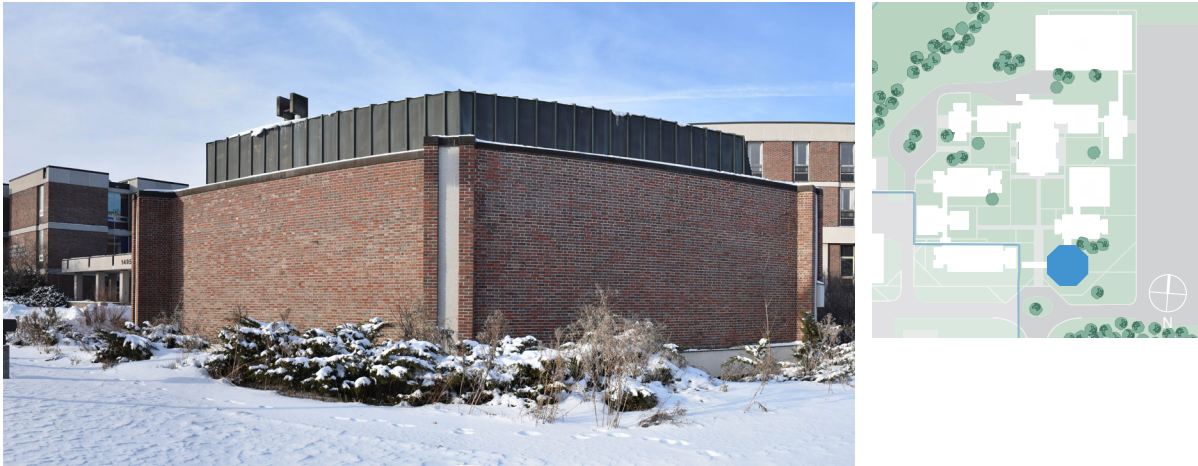
Figure 7. Building F, viewed from southeast (C. Ellis Wong, 2018).
