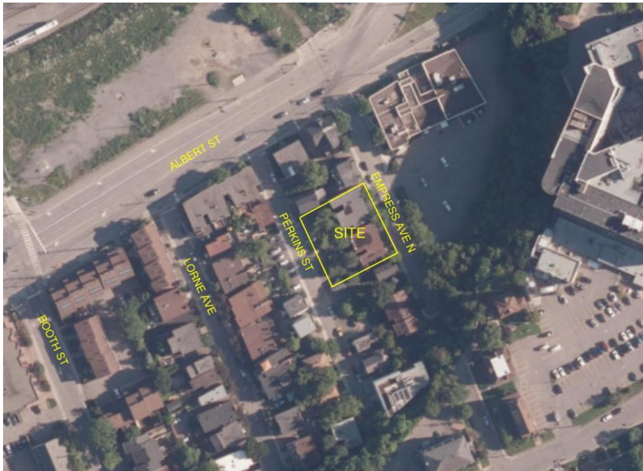
Figure 1 – Aerial View of the Subject Site
