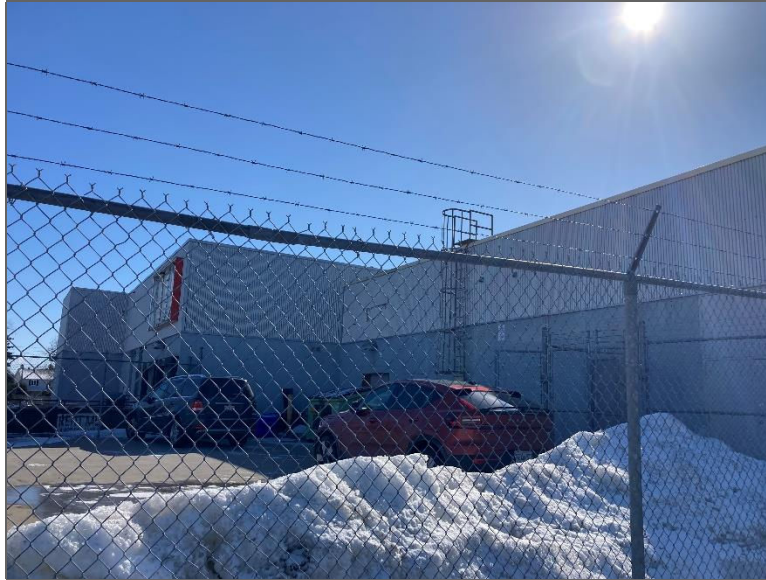
Photo 1 – Site Building (north elevation).
