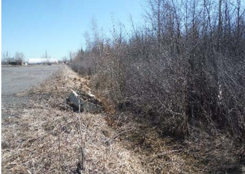
Photo 5: Feature 1b, looking upstream from downstream (April 7, 2020)
