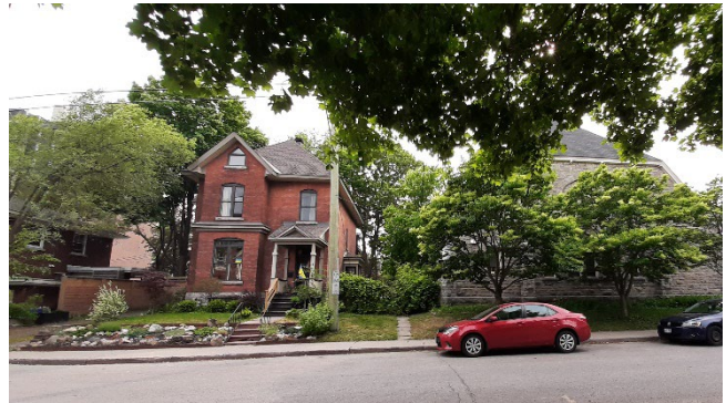
Figure 7: The eastern portion of 321 Chapel Street, looking east from Blackburn Avenue
