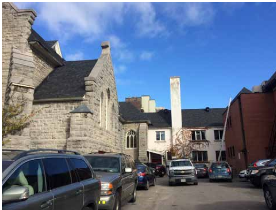
Photograph 2. View, looking east of the parking area and entrance to the Bates Hall, located on the subject property
