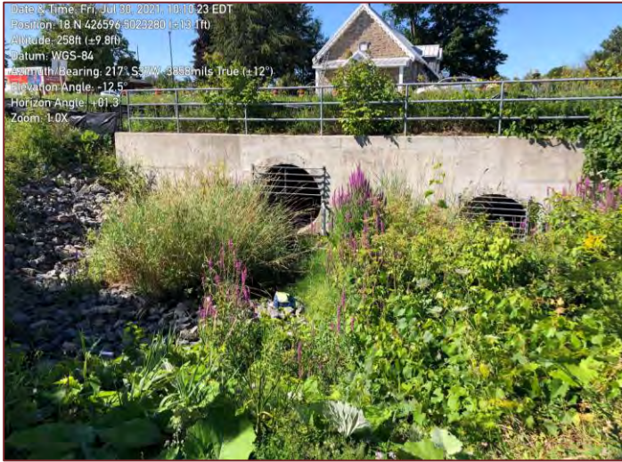
Site Photograph 9 – Inlet for Tributary 4
