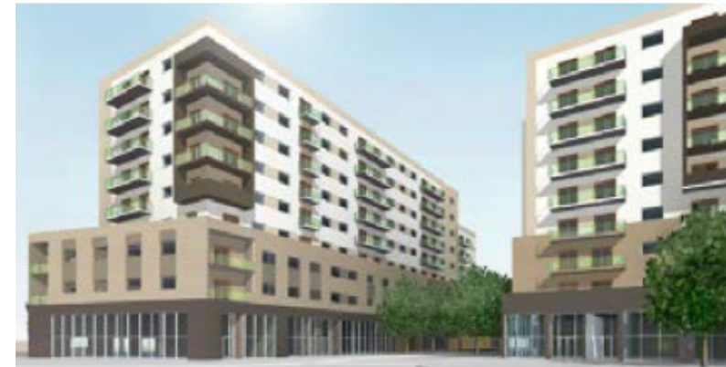
BUILDINGS B AND C FROM HAZELDEAN RD
