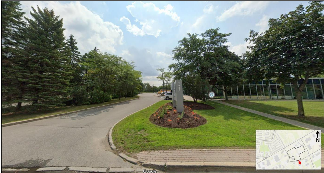
Figure 11: Looking south at the existing office building at 2515 St. Laurent Boulevard
