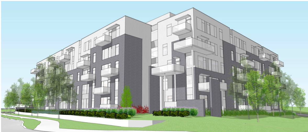
Figure 22: View looking south from Old Carp (Source: Colizza Bruni)
