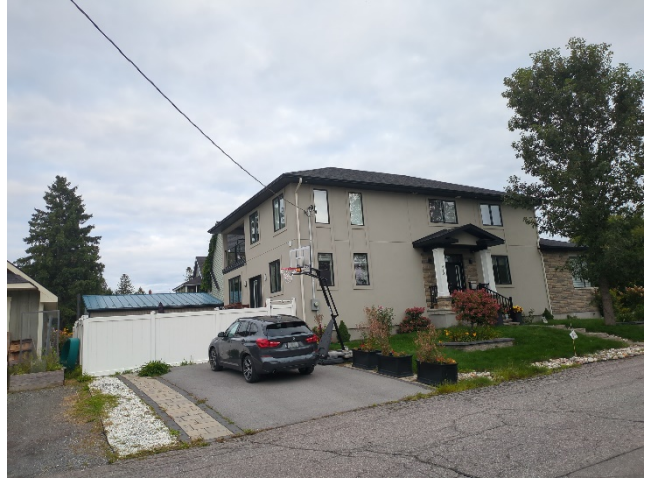
319 Spencer Street, viewed from Rockhurst Road
