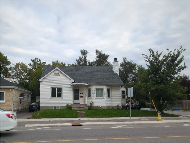
1798 Scott Street, viewed from Scott Street
