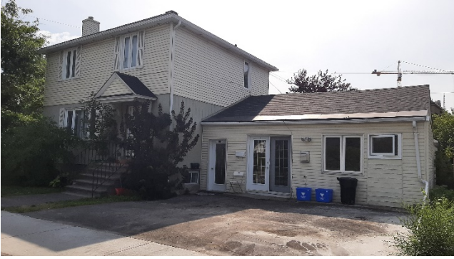
1806 Scott Street, viewed from Scott Street ★
