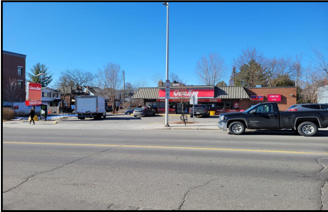
Photograph 3: View of the eastern portion of the Phase I Property, facing west from Bank Street
