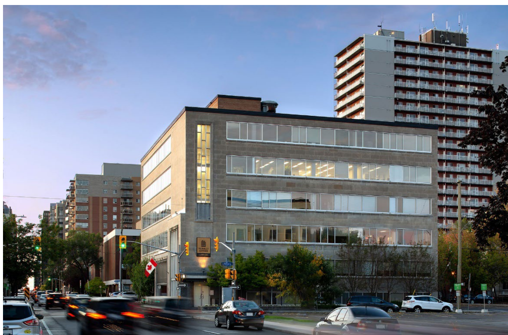
Figure 2.0 – Existing Legion Building at 359 Kent Street.
