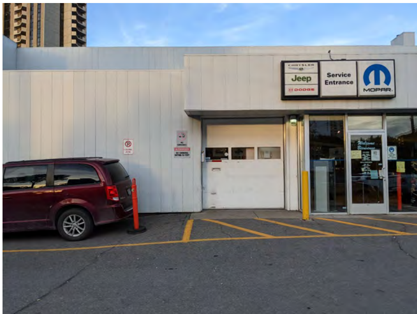
Photo 2 – Service bay entrance, westside of the building
