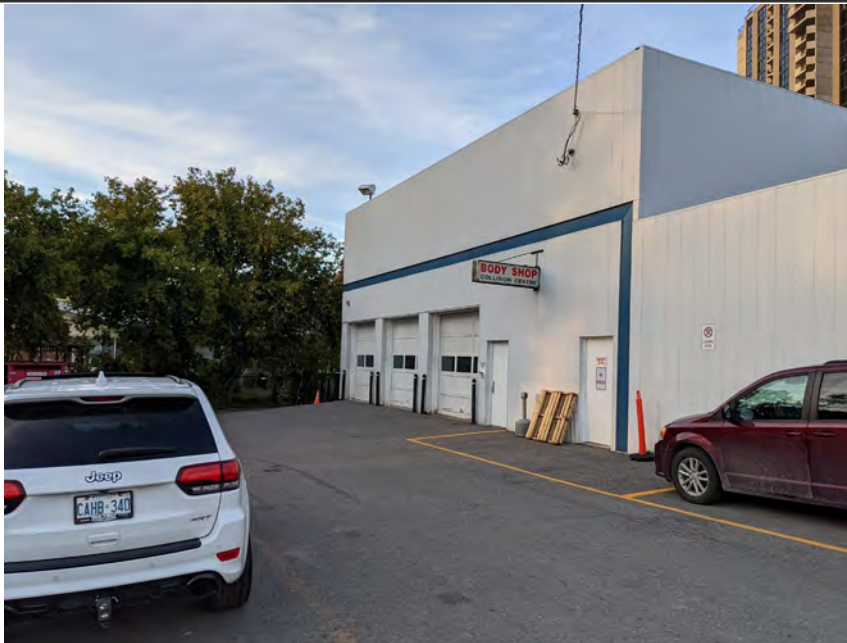
Photo 1 – Body Shop entrance, westside of the building looking north.
