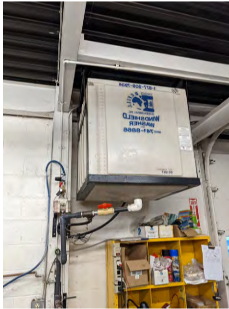
Photo 13 – Washer fluid tote suspended inside the building
