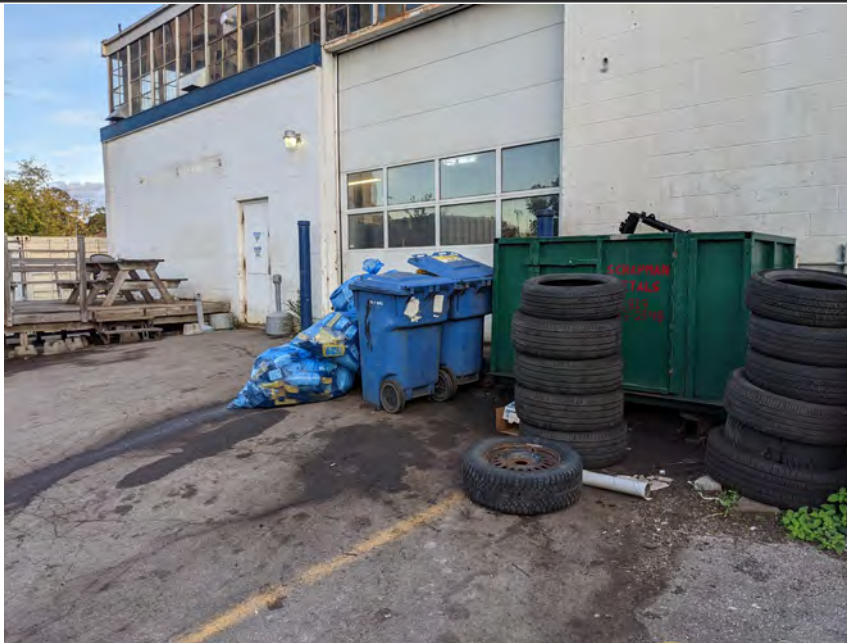
Photo 5 – Garage bay door exit, metal storage bin, oil staining on the pavement, used oil containers, Northside of the building
