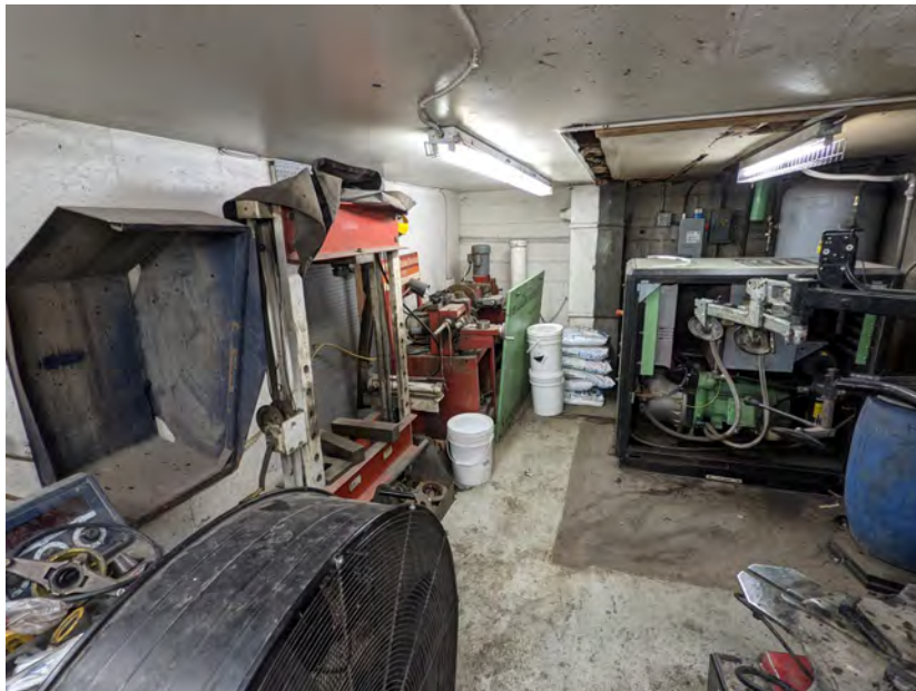
Photo 26 – Compressor and tire balancing room, eastside of the garage
