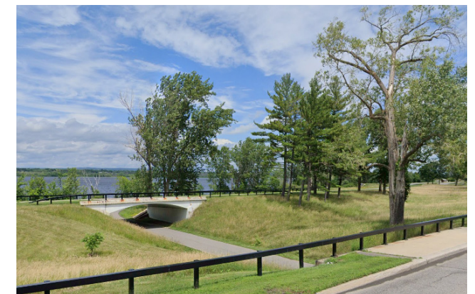
East bound lane, view North towards Ottawa River
