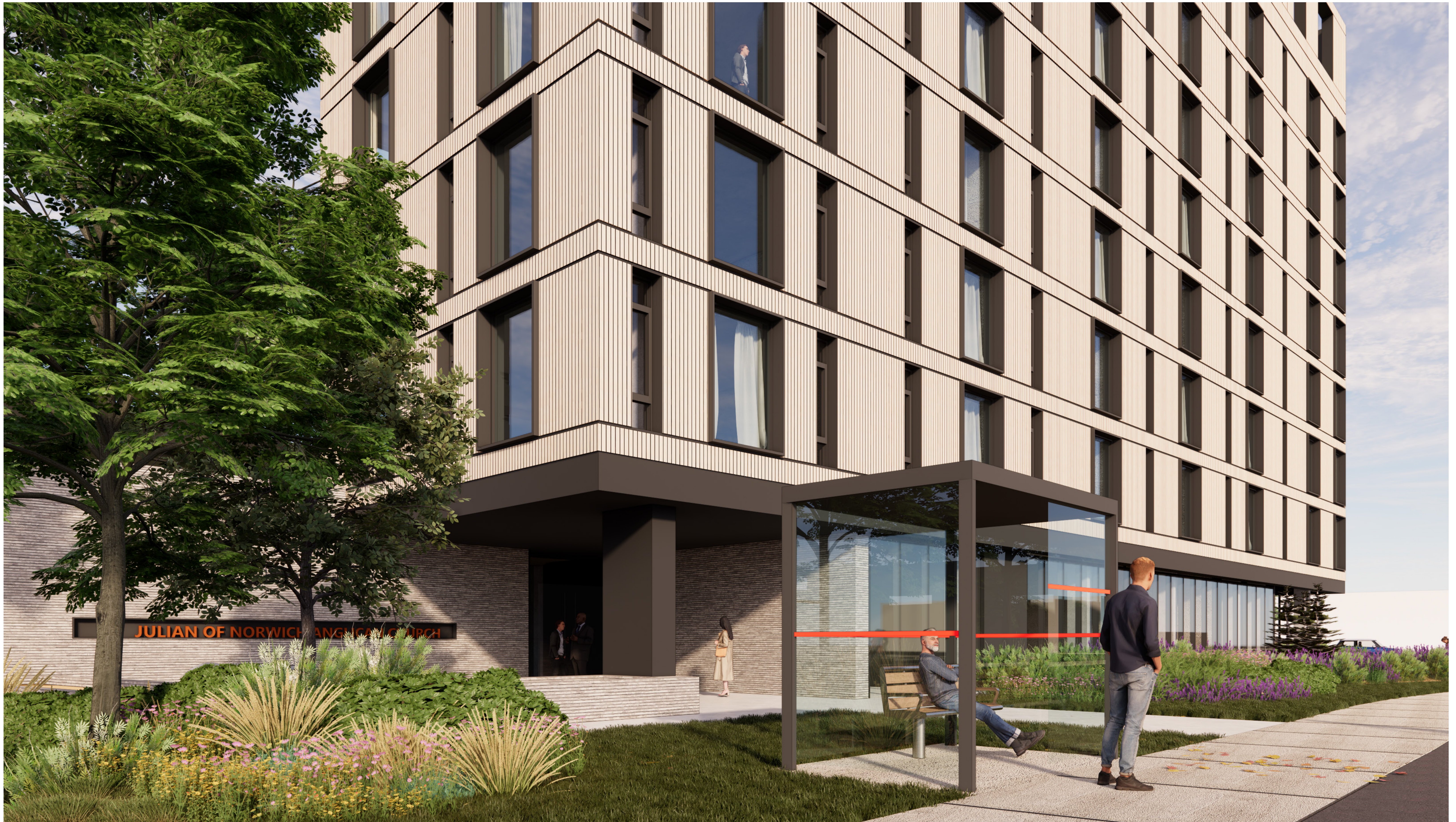
VIEW FROM MERIVALE RD. LOOKING EAST
