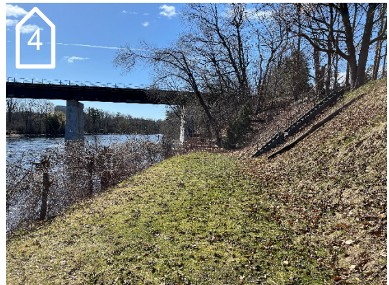
Figure 7: View 4 on key map looking south of the eastern edge of the site.
