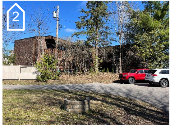
Figure 5: View 2 on key map looking north of the northeastern edge of the subject site.
