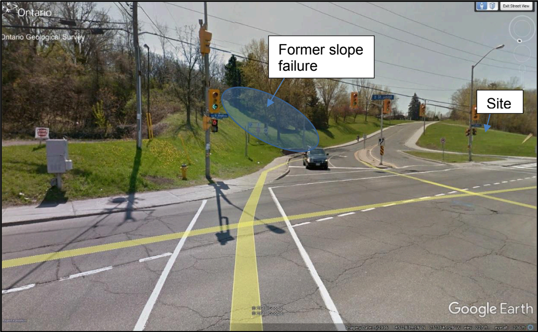
Photo 5: Area of former slope failure noted in Photos 1 and 2. Subject site is property along the right side of the photograph.
