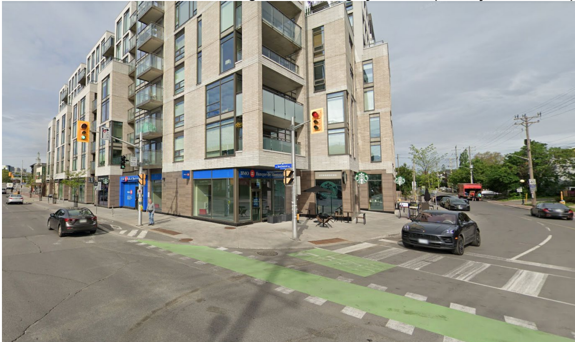
Figure 21: Existing Cycle Track (MacKay / Beechwood)
