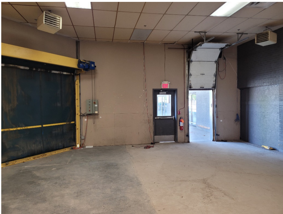
Photograph 8: View of interior of the shipping and receiving area in the northwest portion of the Site building.
