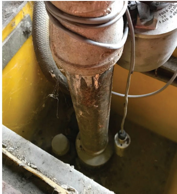
SENSOR LOCATED BENEATH DISPENSER
