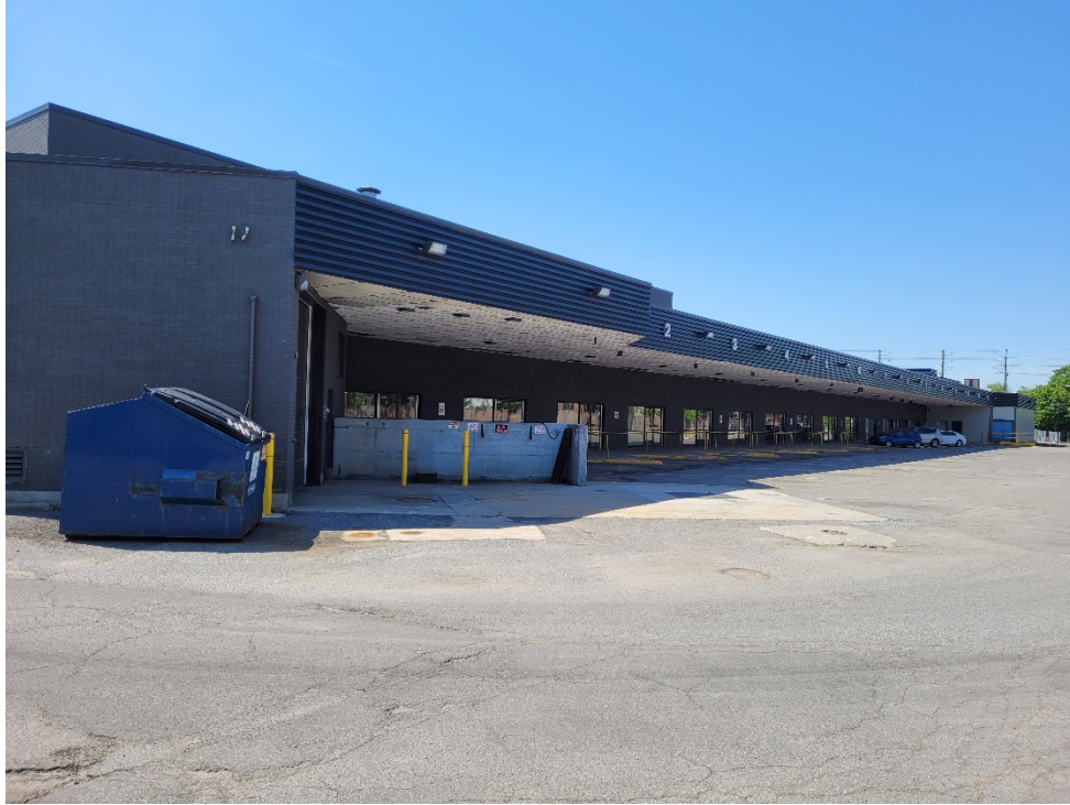
Photograph 3: View of the north side of the Phase One Property looking west. View shows the terminals for the former central bus station. The diesel underground storage tank and former fueling area is visible in this photograph.
