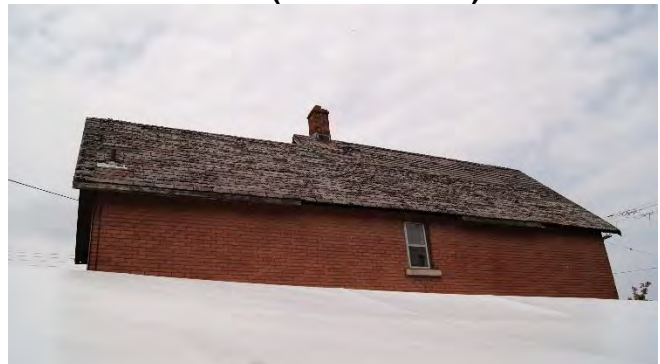
Roof (view from south)
