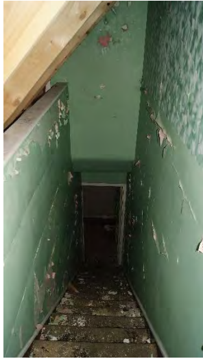
Stairs to basement
