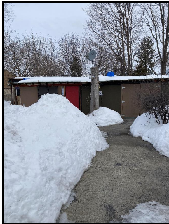
Photograph 2: View of the outbuilding on the 1184 Cummings Avenue property, facing north.
