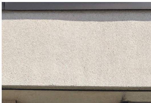
Figure 23. Aggregate-faced concrete paneling (ERA, 2021).
