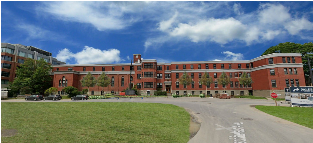
Figure 16. View from des Oblats Avenue
