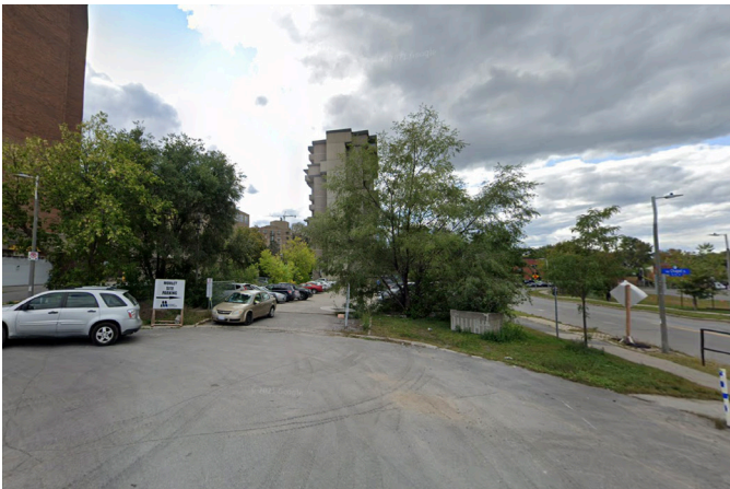
Chapel Street Frontage showing existing parkade.
