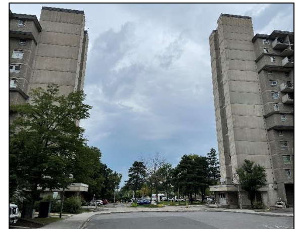
Figure 2-15: Friel Street looking north towards 200 and 201 Friel Street
