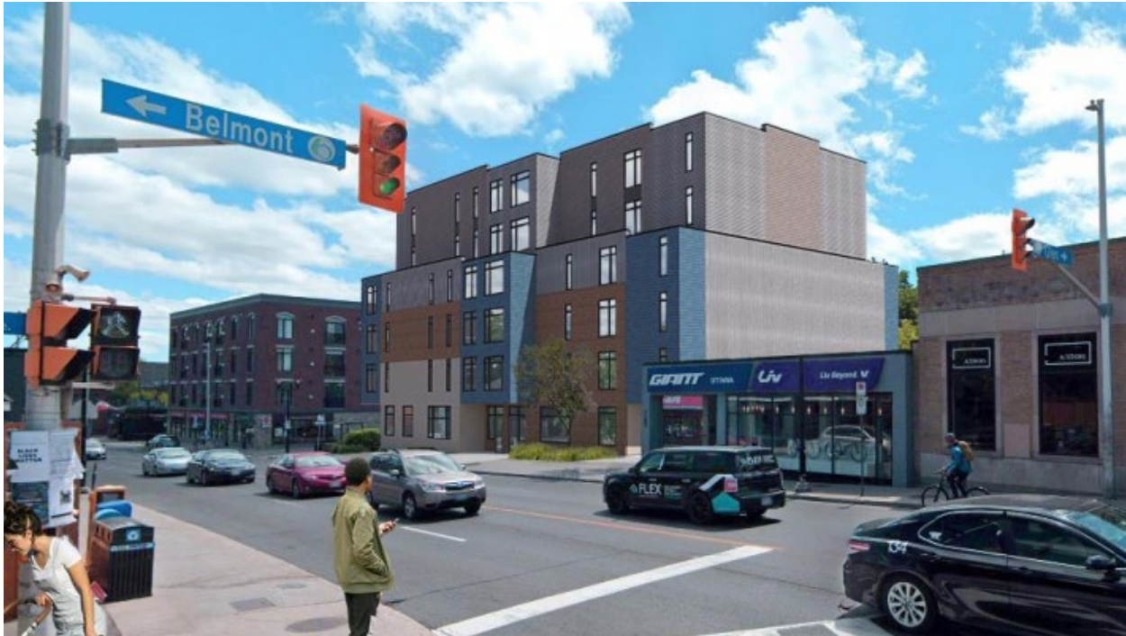
Figure 14: View of Building Looking South (Bank Street)
