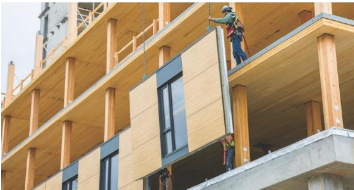
CROSS LAMINATED CONSTRUCTION, BROCK COMMONS, UBC
