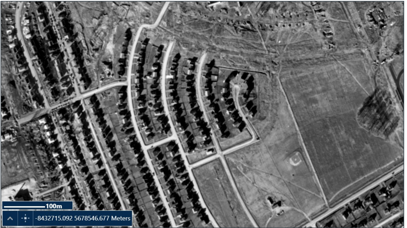
A1 - Aerial Photograph 1958 (GeoOttawa).
