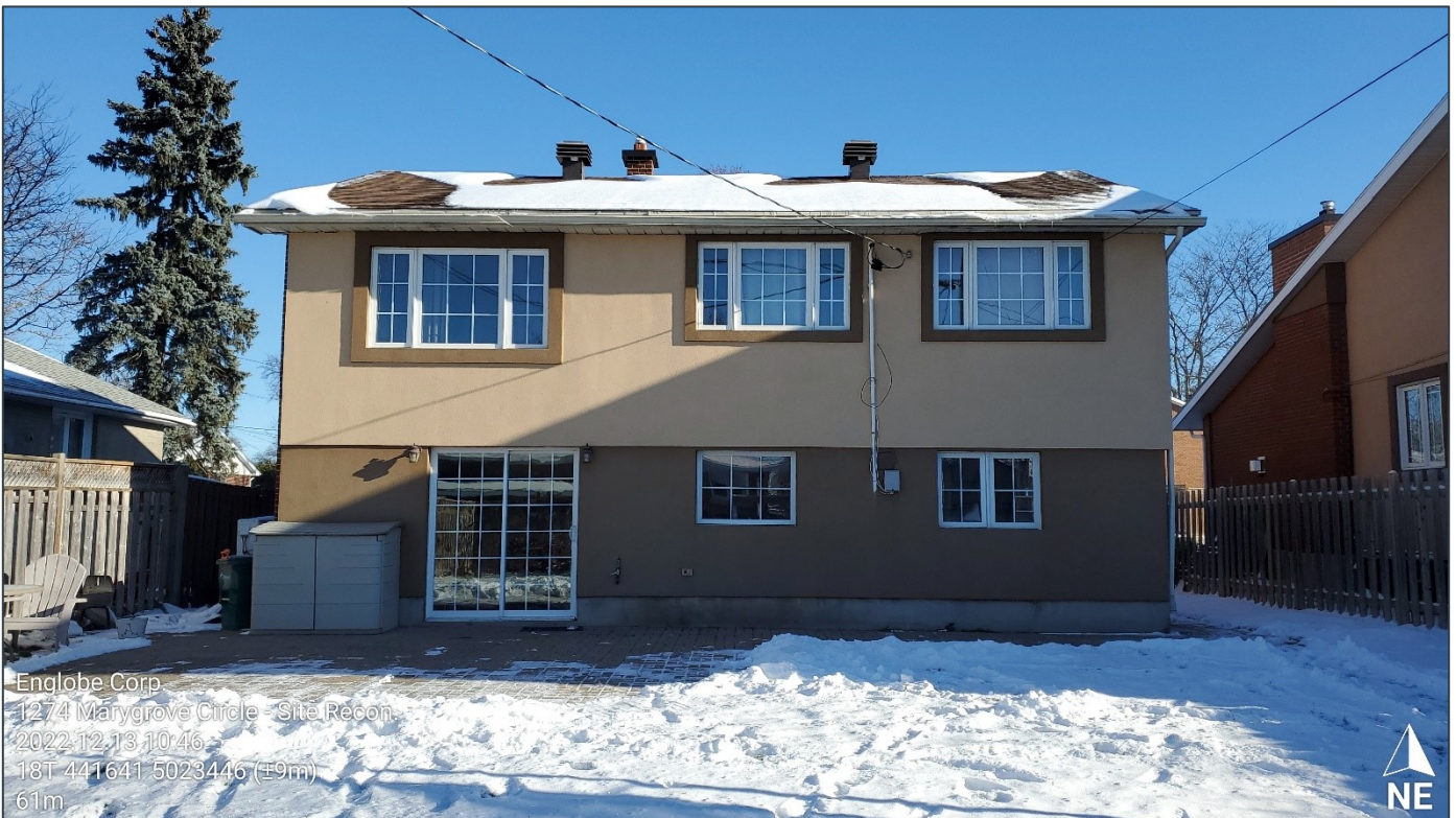
Site Photograph 2: Overview of rear face of 1274 Marygrove Circle.
