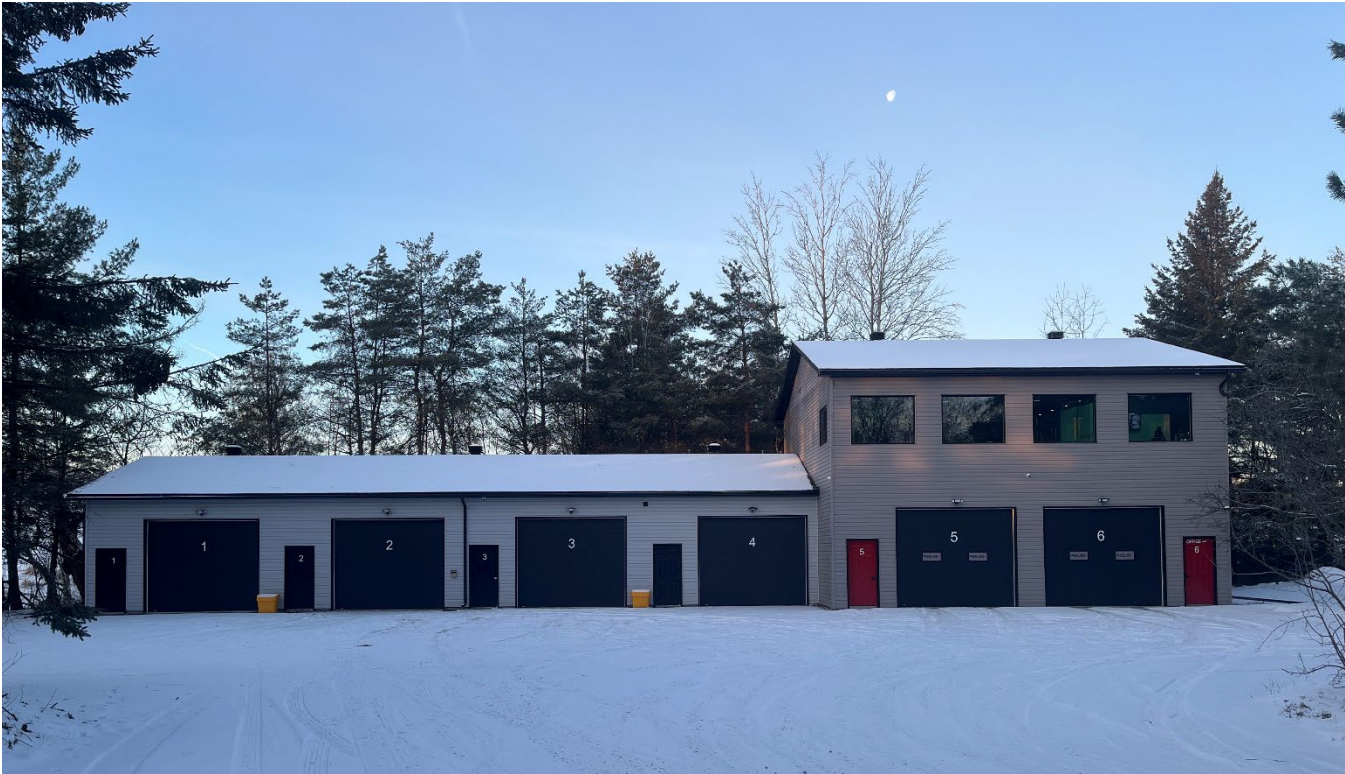
Figure 8. Recently constructed building that is associated with a contractor’s business, with 6 individual warehouse bays and second storey office
