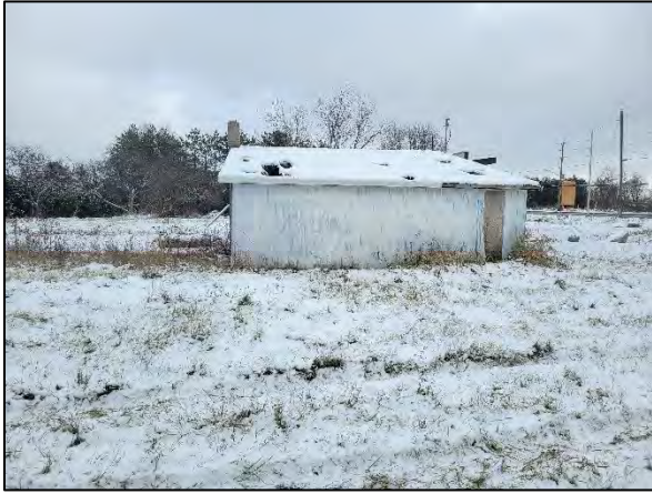
7. Photo is taken facing east from the west side of the garage building on 3493 Innes Road.
