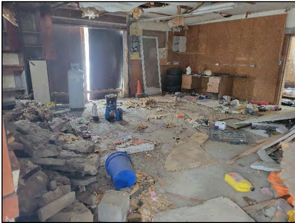
4. Photo is taken inside the garage structure at 3493 Innes Road.
