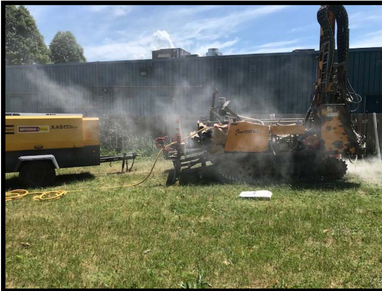
Drilling at MW2 – June 19, 2020
