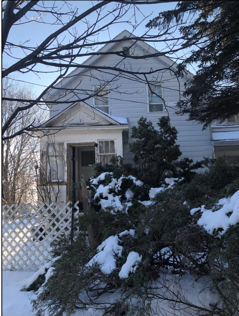
Photo 3: East of the residential dwelling, facing towards the west building face.
