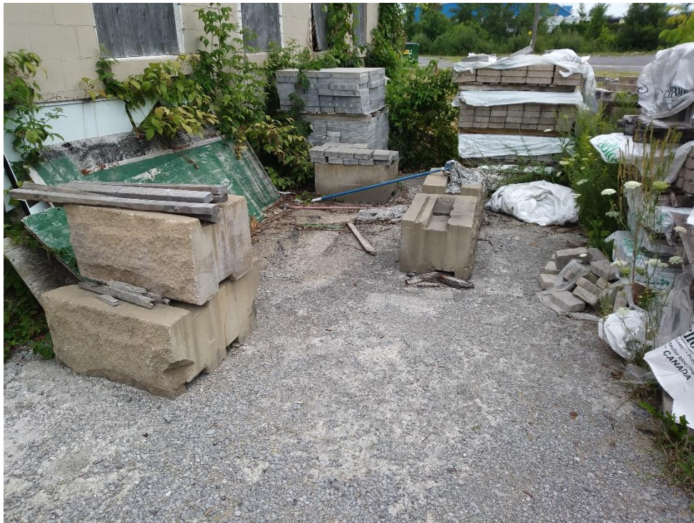
Photo 5: Location of former above ground diesel fuel storage tank, rear of garage facing northeast.
