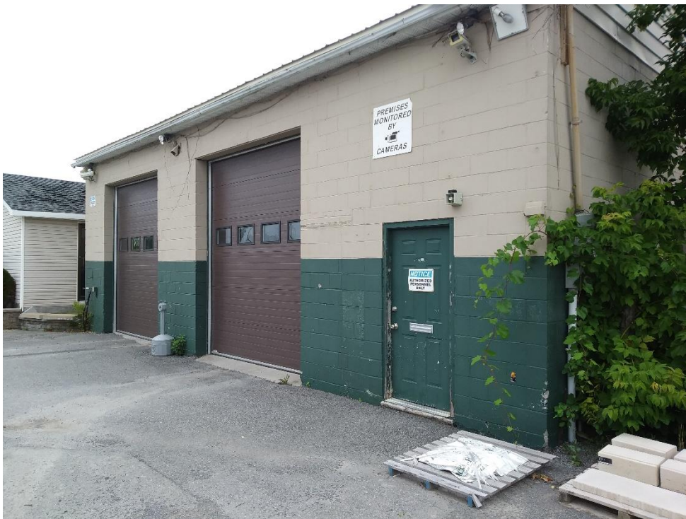
Photo 2: Former RV automotive garage, facing northeast.
