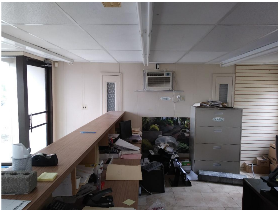
Photo 6: Interior of office building
