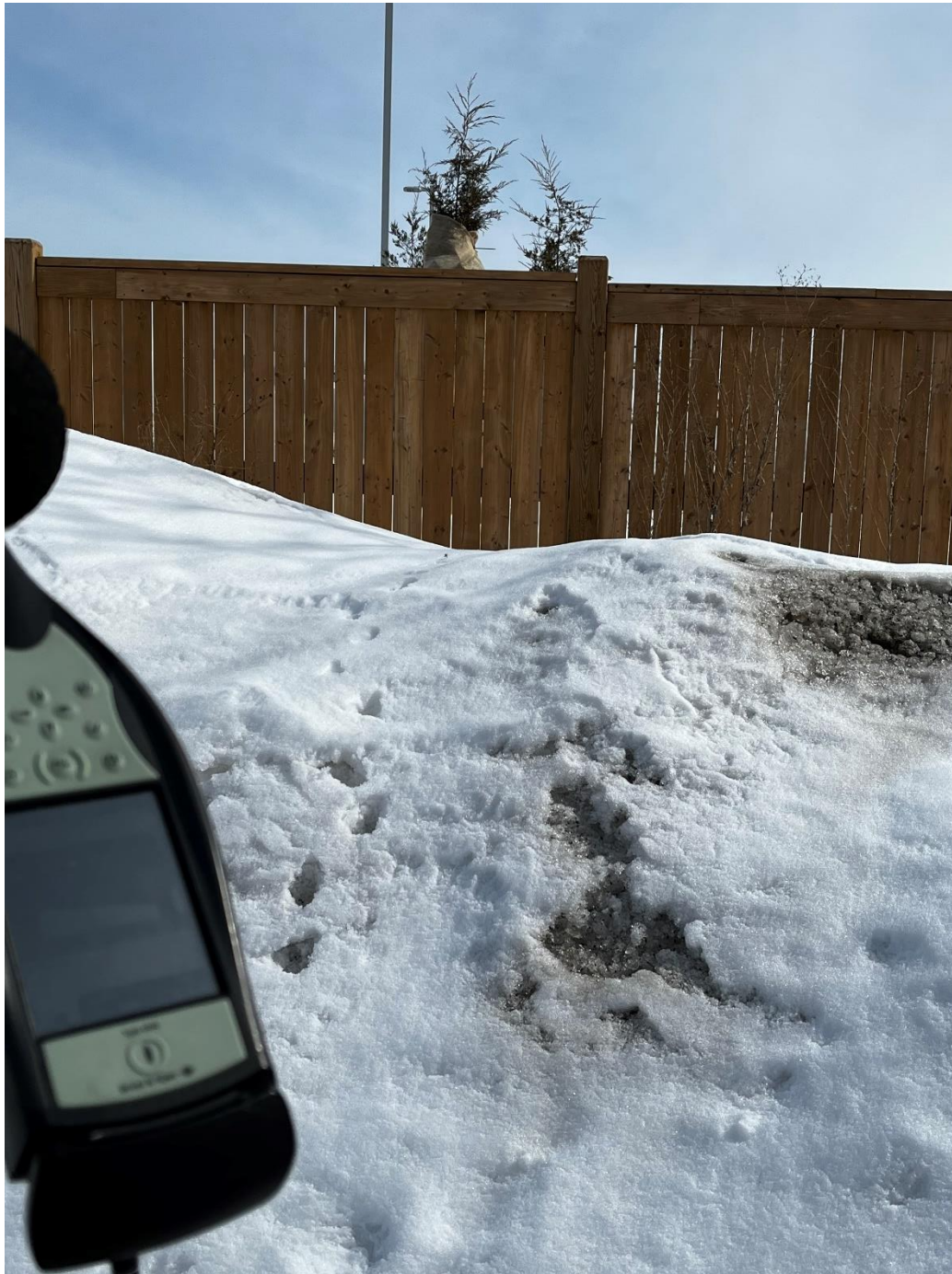
PHOTOGRAPH 5: EXISTING PERIMETER FENCE GAPS BETWEEN WOOD PLANKS
