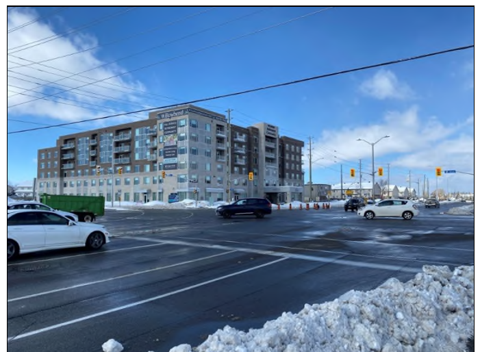
6. 1980 Trim Road – Willowbend Retirement Community building located to the northwest of the Site.
