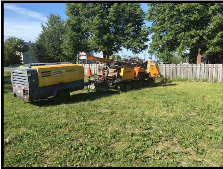
Drill Setting Up at MW1 – June 19, 2020
