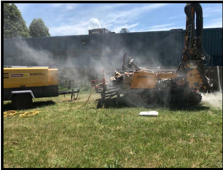
Drilling at MW2 – June 19, 2020
