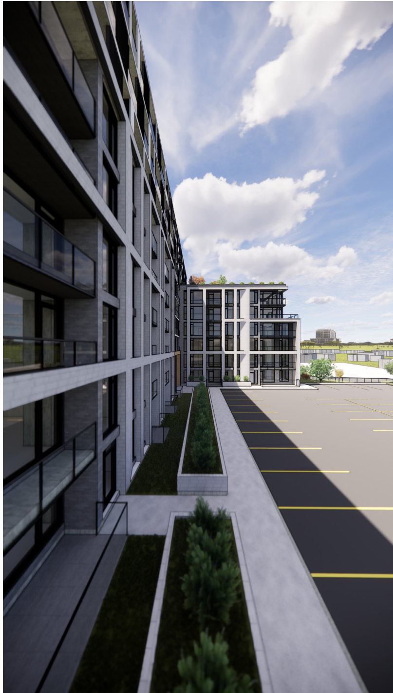
View of Apartment Building and Podium Planters
