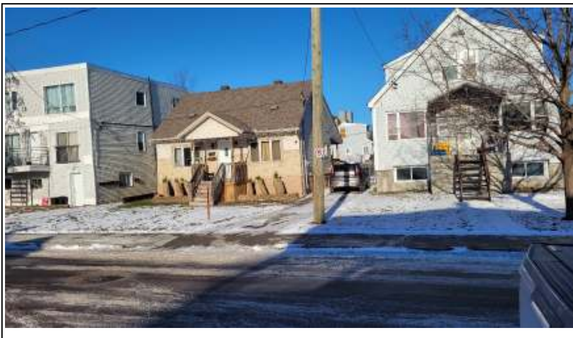
Photograph 10: View north-east from south side of Ste-Cecile Street with front (south) side of 73 Ste-Cecile in photo center and 79 Ste-Cecile on left. Sanitary sewer manhole in center of Ste-Cecile Street in front of 73 Ste-Cecile.
