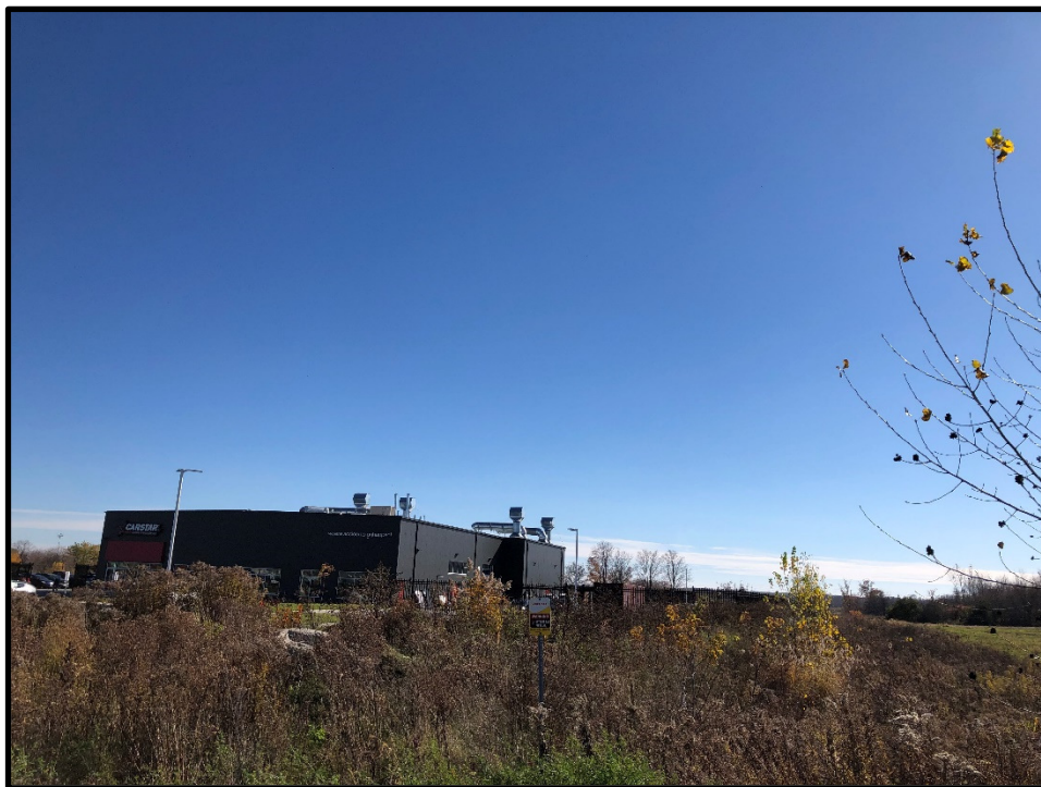
Photograph 6: View of the adjacent automotive service shop on Dealership Drive (Site 2), looking south from Dealership Drive.
