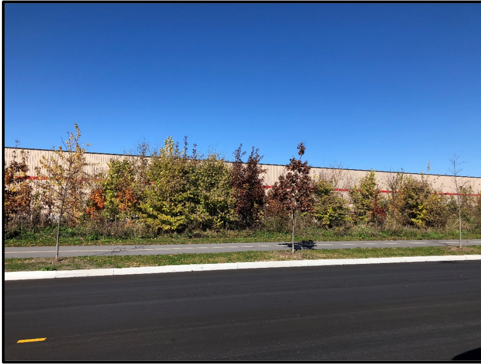
Photograph 3: Commercial property (Costco) located to the north of 444 Citigate Drive (Site 1), looking to the north from Systemhouse Street.
