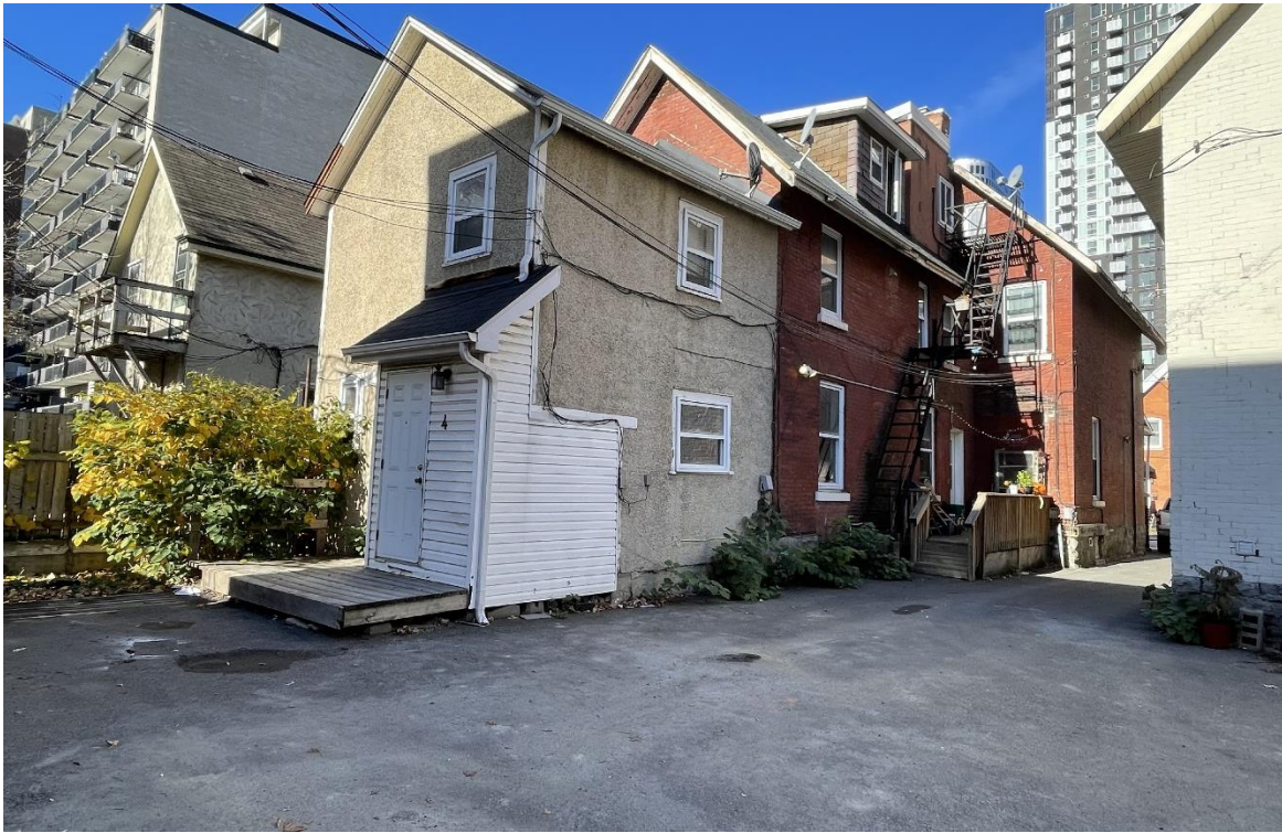
Photograph 3: View of the 232 Lisgar Street, looking northwest.
