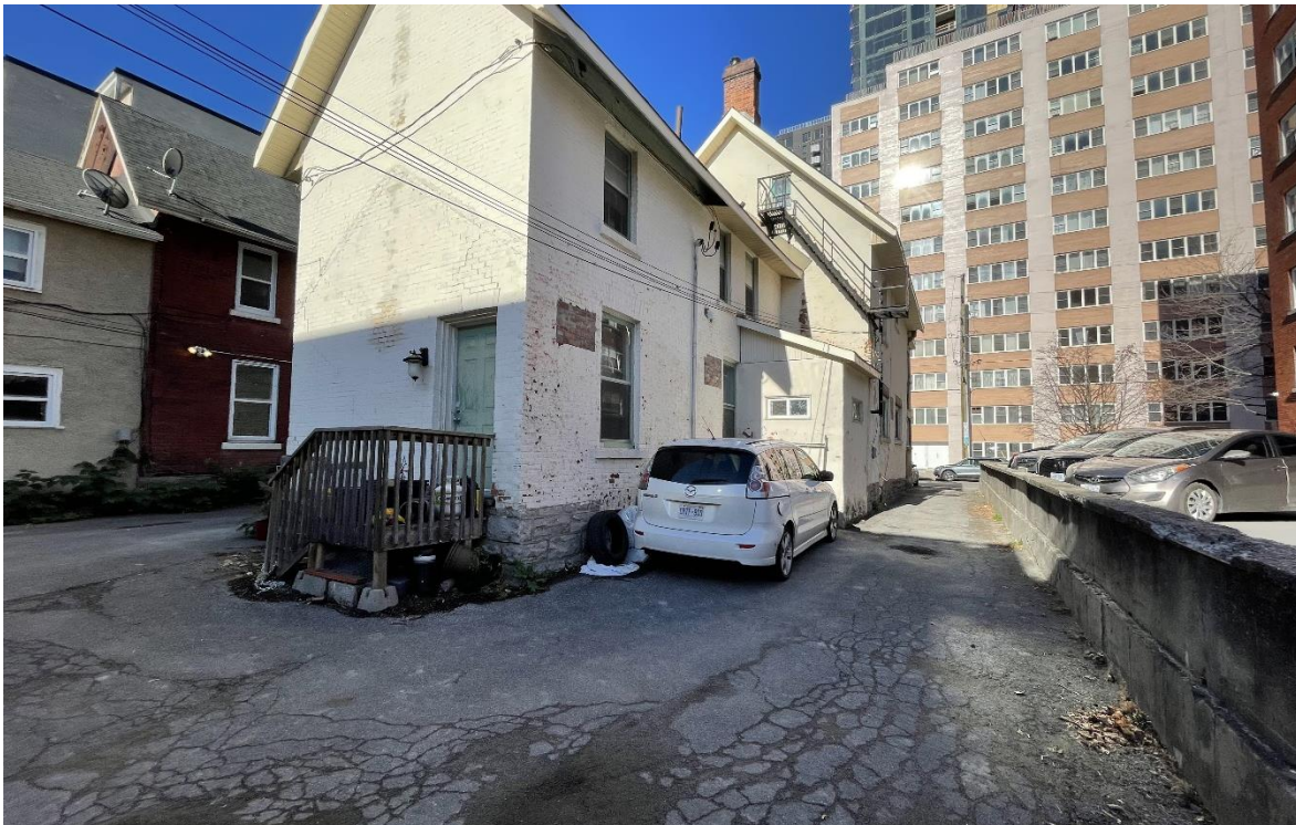
Photograph 4: View of the 230 Lisgar Street, looking northwest
