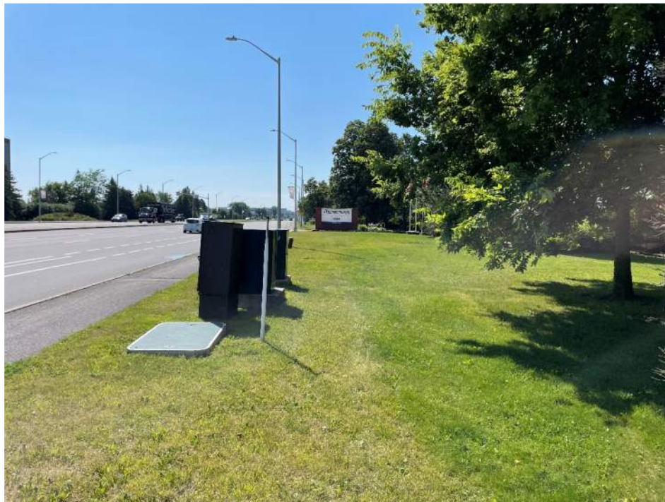
Photo 2: Northern corner of the phase one property looking southeast along property line. Communication pedestals lined up along the side of March Road.
