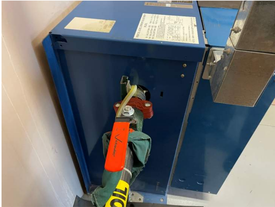
Photo 7: Hydraulic oil storage tank and pump for elevator system in 603 March Road.
