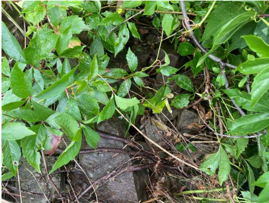
Photo 17: Broken rock fill observed on the phase one property at the corner of Hines Road.
