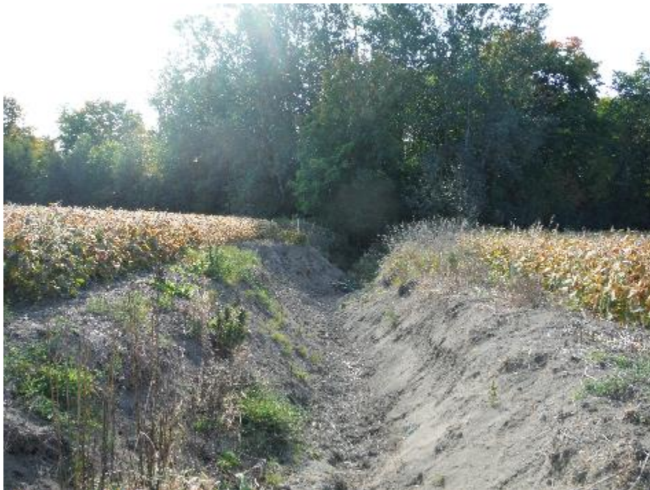
Photo 3: North Channel, downstream of the reach break B (September 21, 2020)
