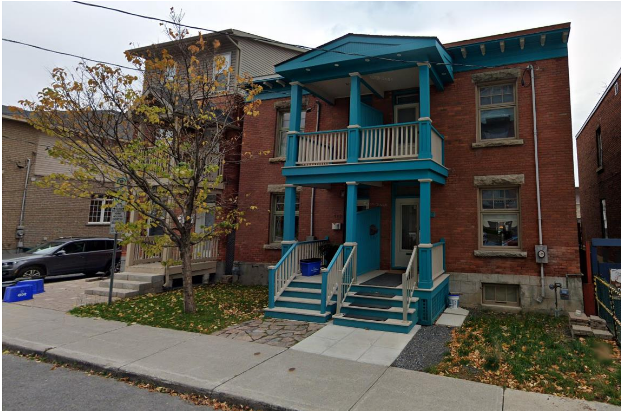
Figure 5: Semi-Detached Dwelling to the North of the Subject Site
