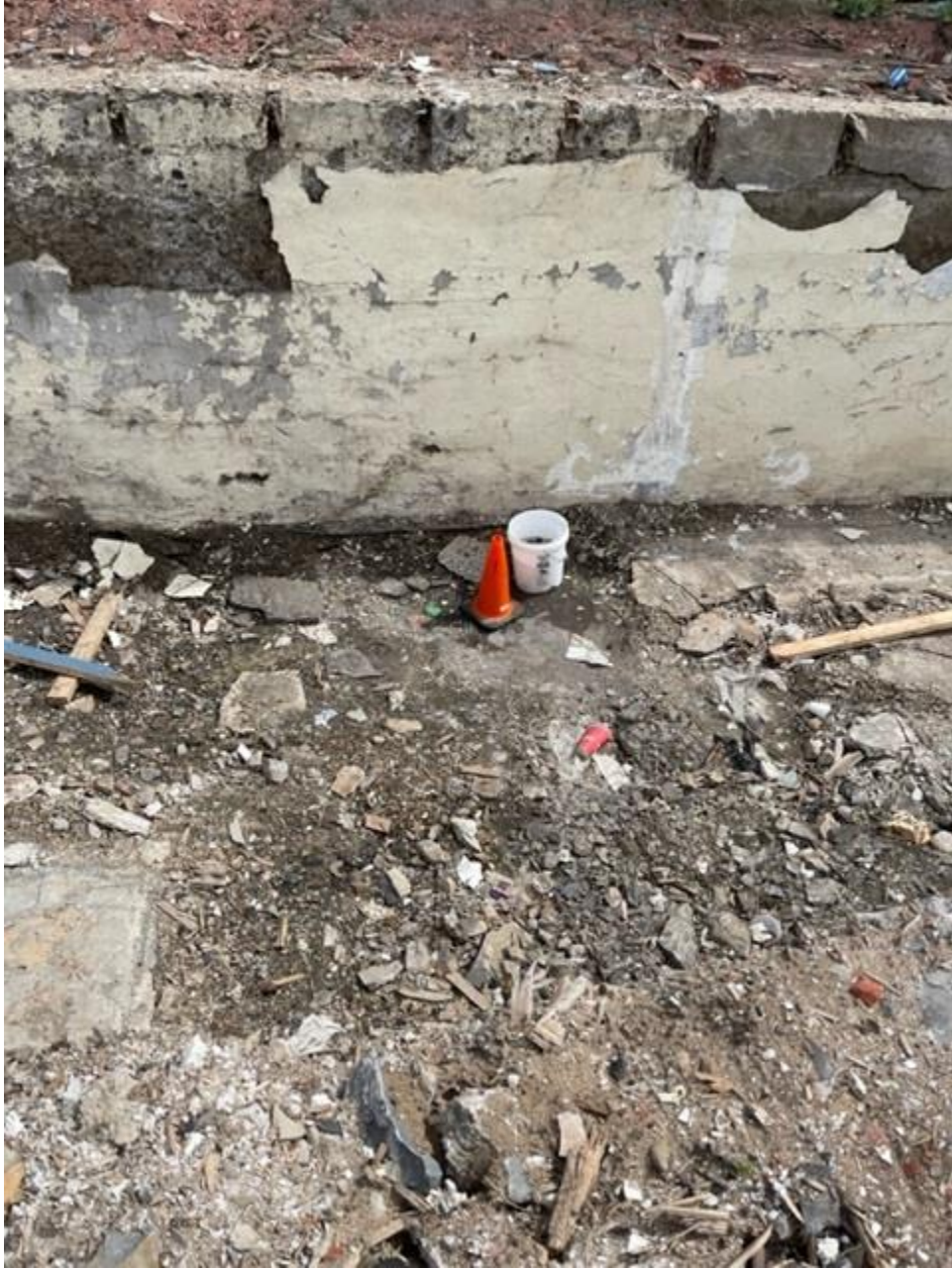
Image 5 – EX–MW1 within basement foundation southwest of the subject property
